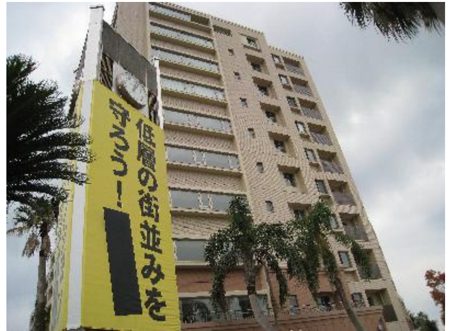
A case of conflict of a condo building in Fukuoka
