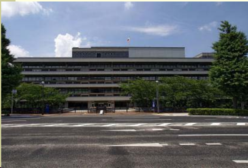
Main Library in Nagatacho, Tokyo
