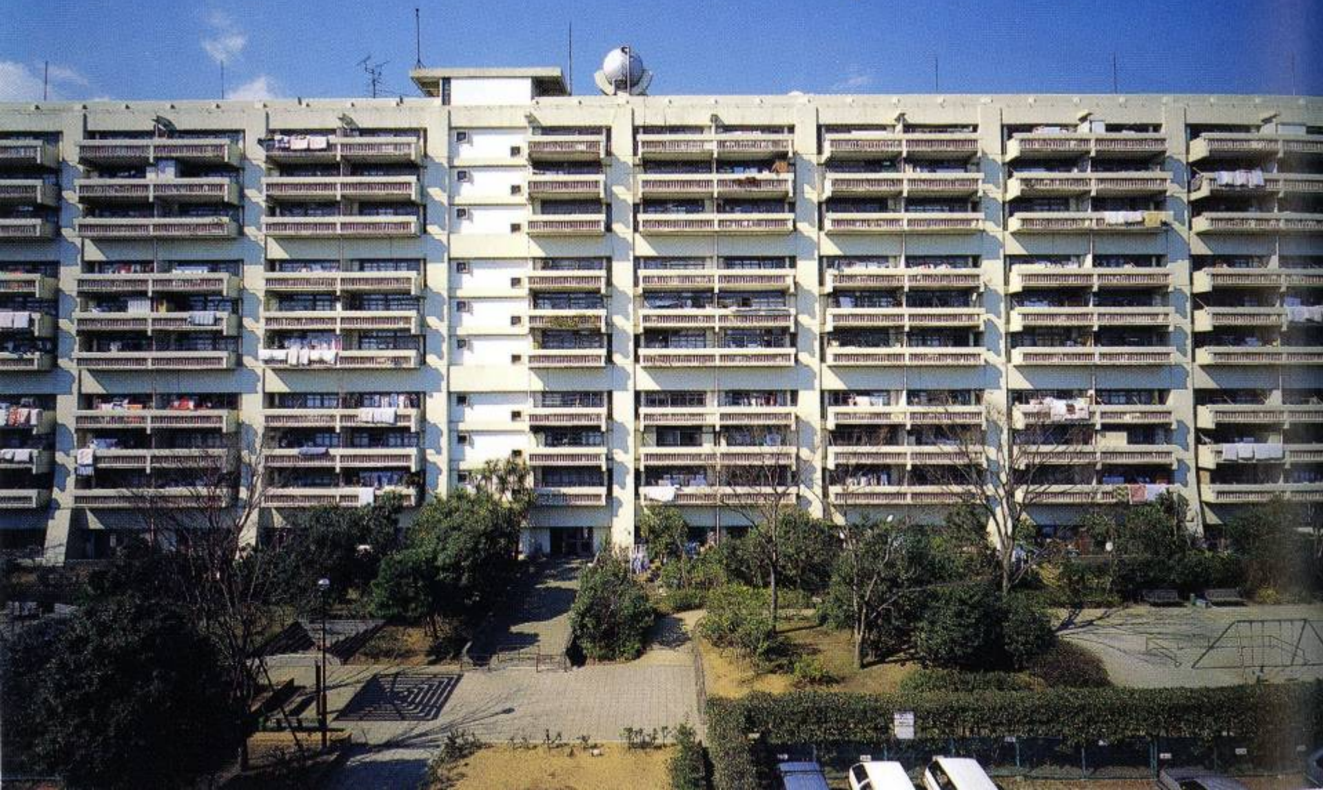
Harumi Apartment House (1958-2003)
